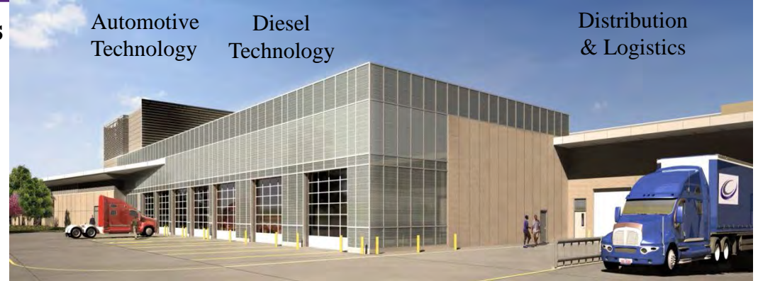
Exterior View from Southeast
