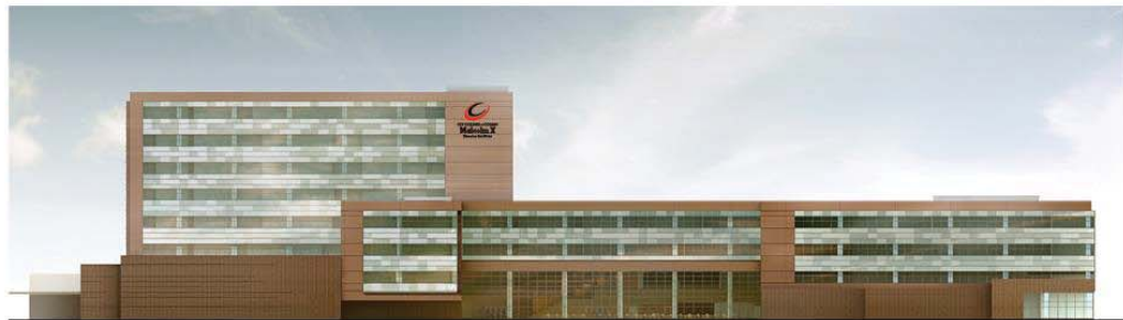
North Elevation (Illuminated)
