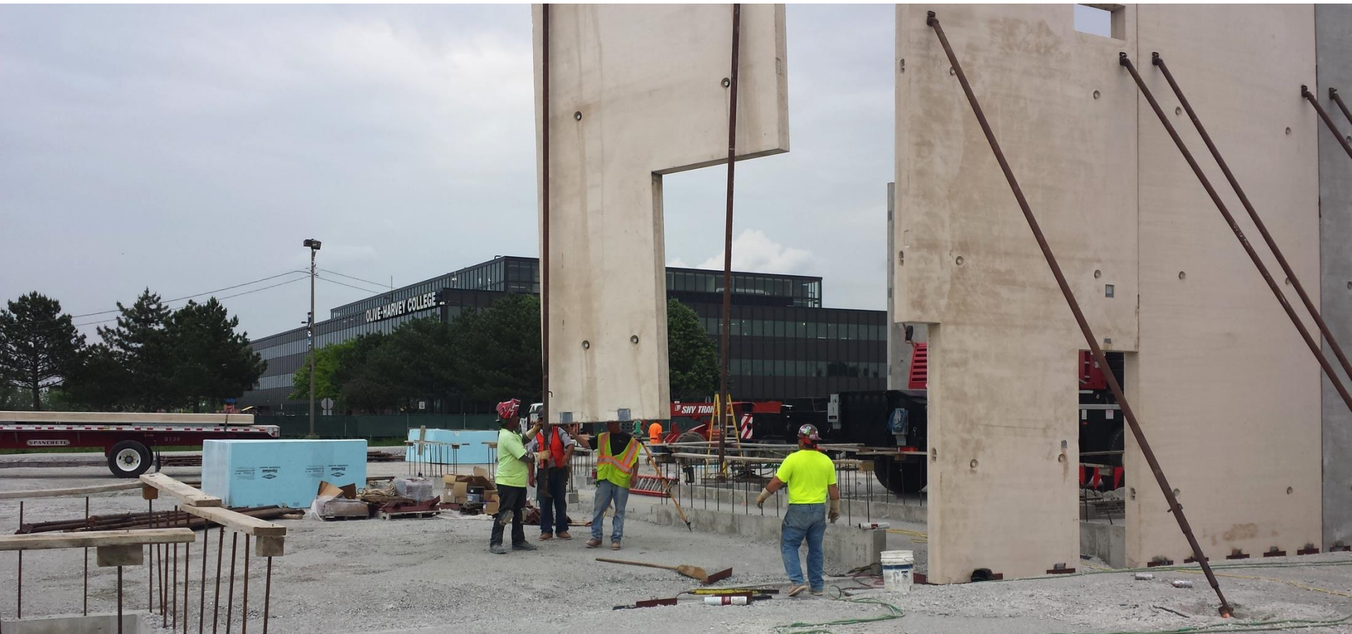
Installation of precast concrete panels near the diesel engine labs
