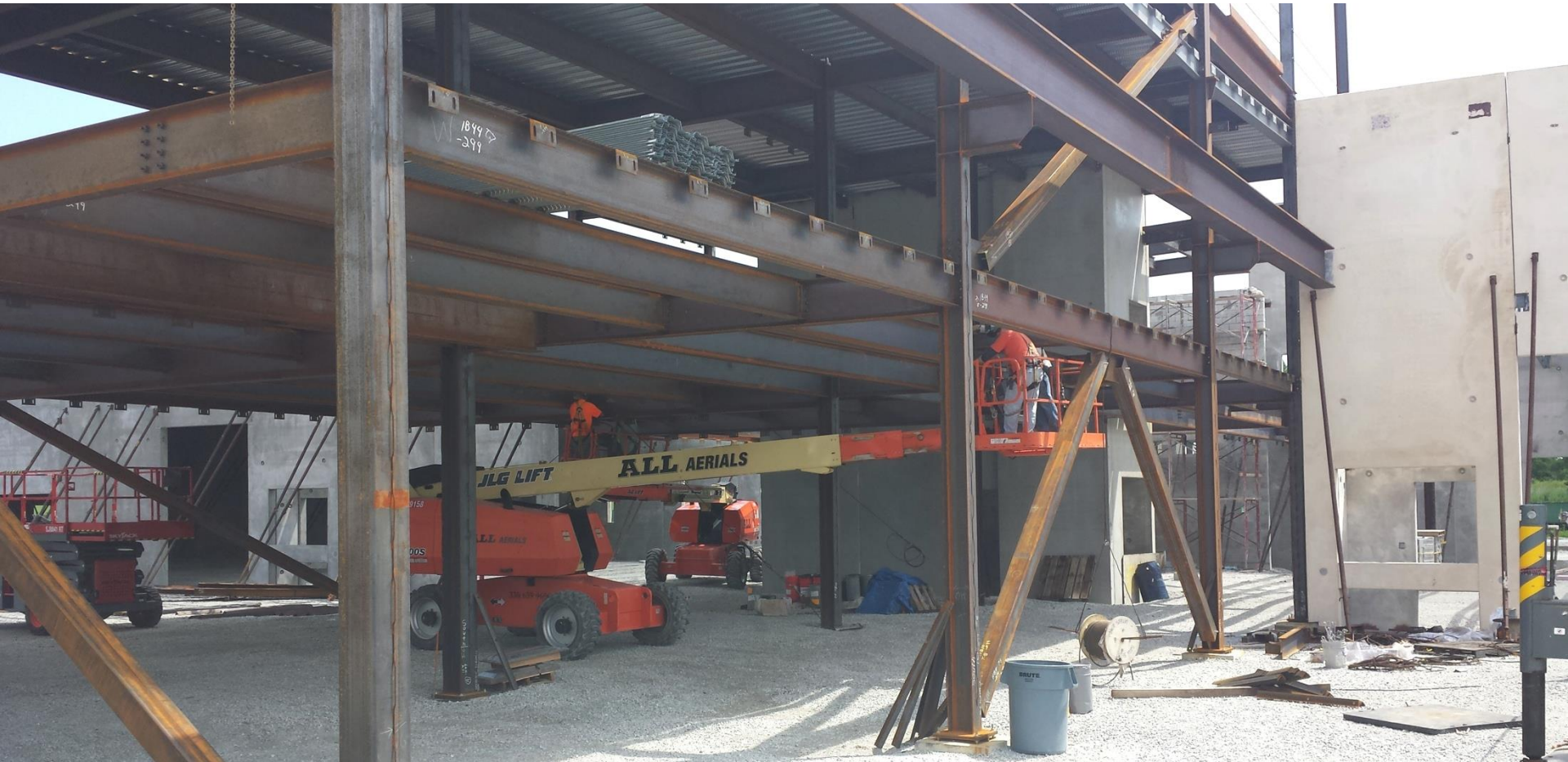
Installation of steel within the auto and diesel lab areas
