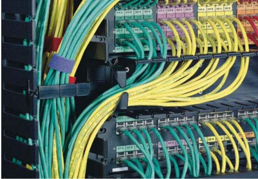
Figure 11 : Example of properly dressed cables
